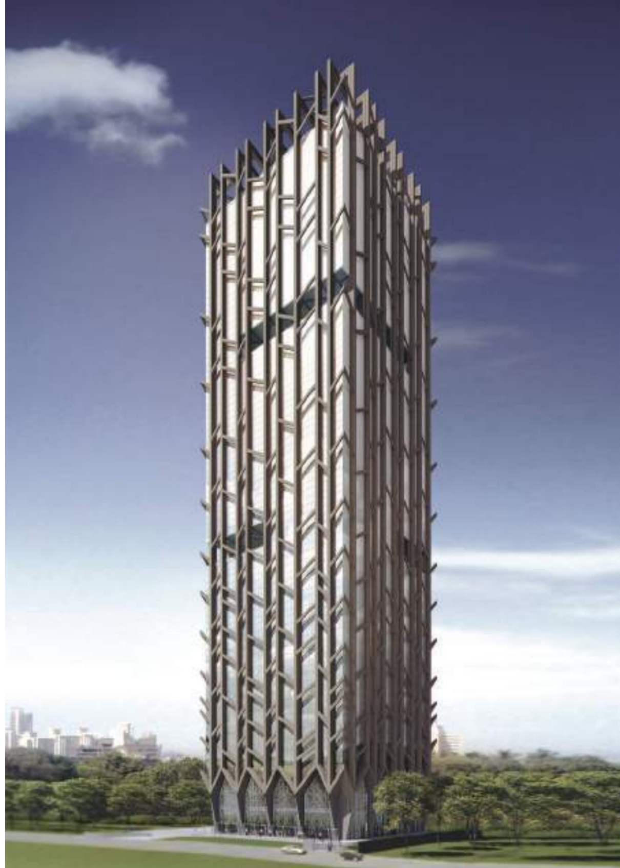
Branching tree structure façade of the iconic commercial tower
